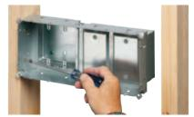
2 Or attach to a wood stud using #6 screws. Pull wires.
