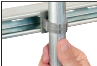
5 Secure installation of conduit to strut.
