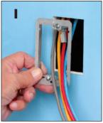
Trace bracket along inside of bracket. Cut hole along outside of line. Pull wires.
