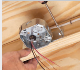
FBS415S/FBS420S Mount on SIDE of Joist
